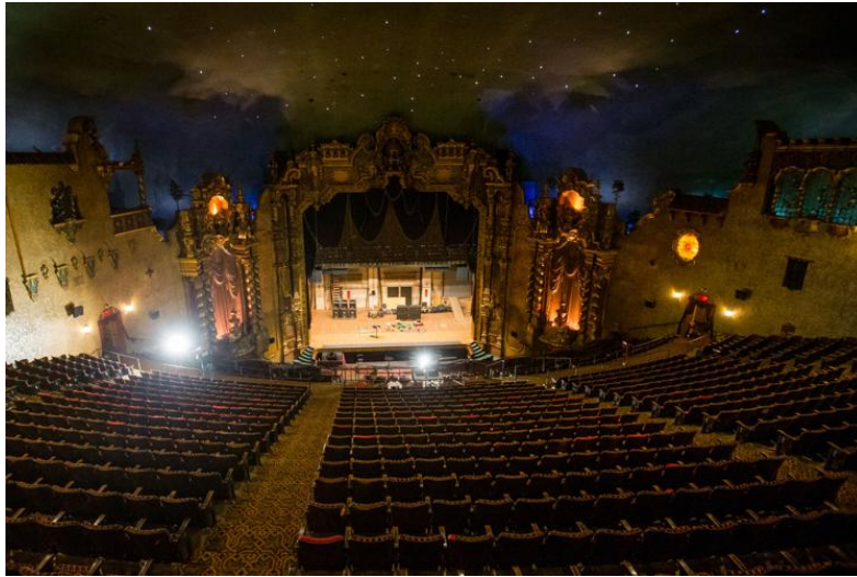
Renovations continue at the Keith-Albee Performing Arts Center on Tuesday, Aug. 18, 2020, in Huntington. Sholten Singer/The Herald-Dispatch
